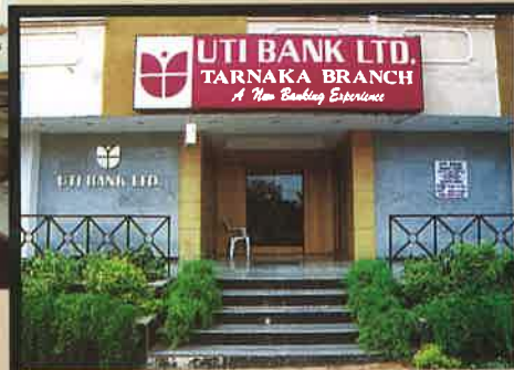
Tarnaka Branch (Andhra Pradesh)
